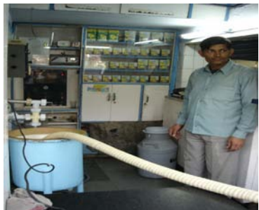
Chilled, pasteurized milk being pumped into a tank at the outlet.
